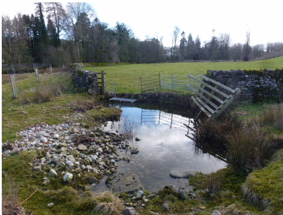
010 – Watergate needs replaced and washed out area reinstated
