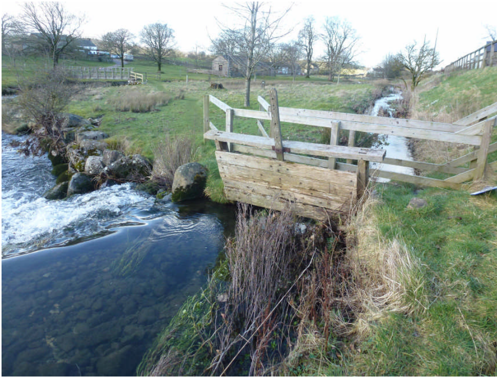
004 / 005 Mill race sluice gate needs replaced
