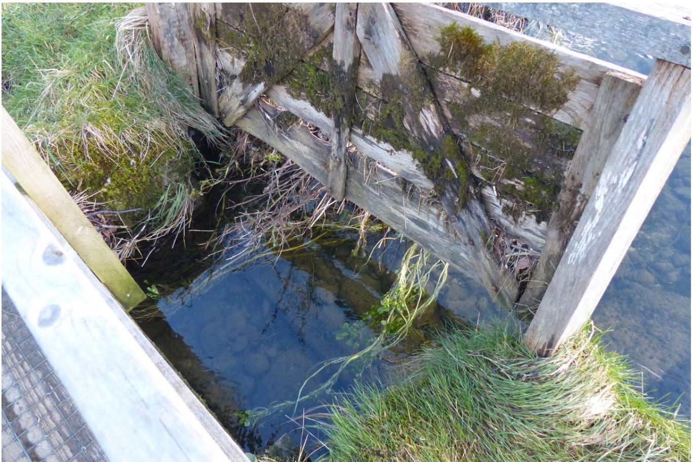
004 / 005 Mill race sluice gate needs replaced
