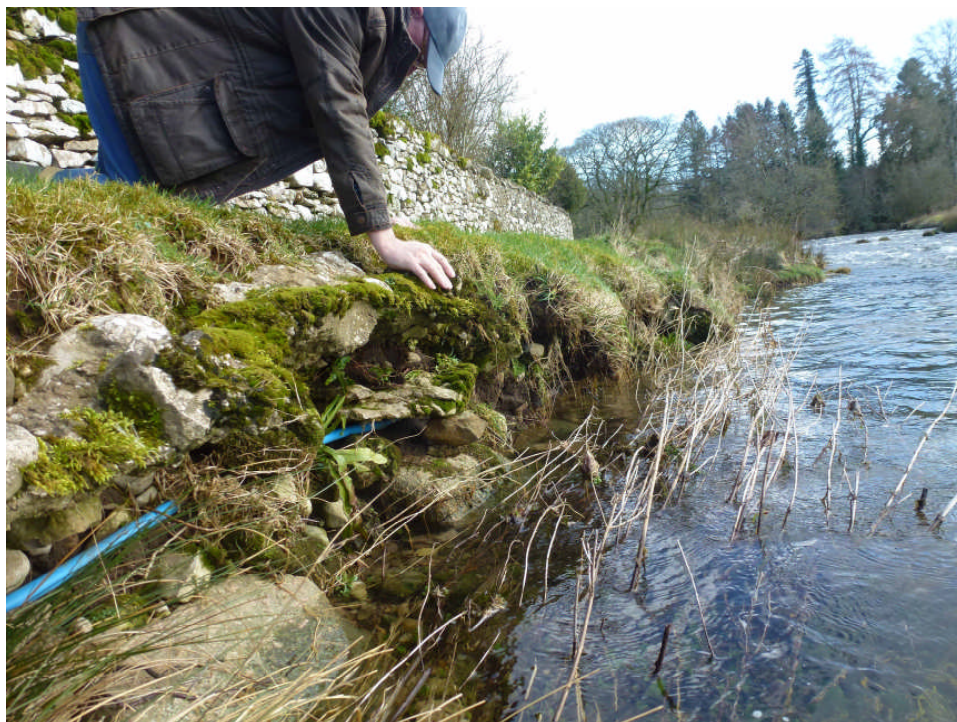
012 – Undercutting footpath edge + exposed water supply pipe
